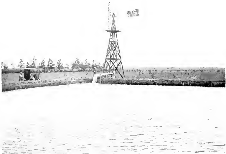
A TYPICAL PRAIRIE IRRIGATION PLANT. FILLING D. M. FROST'S RESERVOIR, GARDEN CITY, KANSAS.
